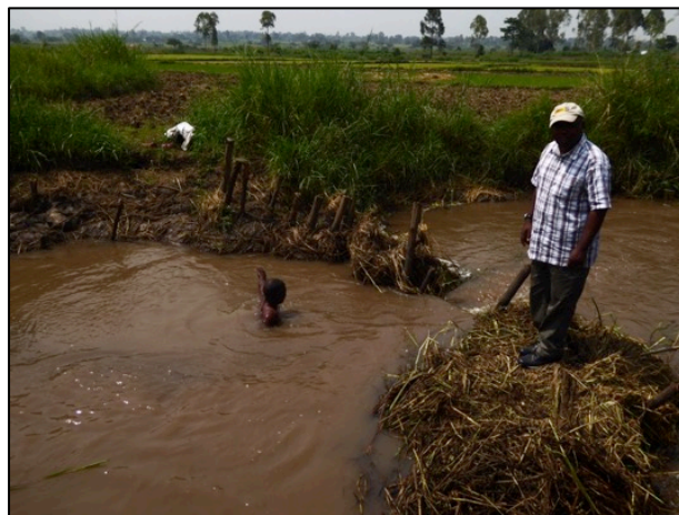
Figure 3: dam to divert water for dry season storage
